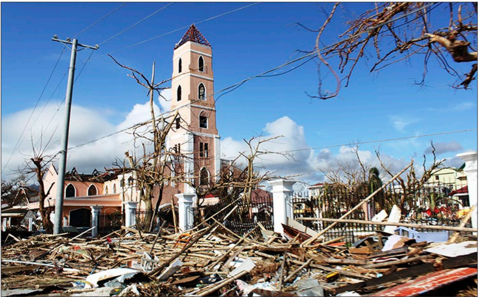
Santo Niño Church survived. The structure was safe for people to shelter there.
